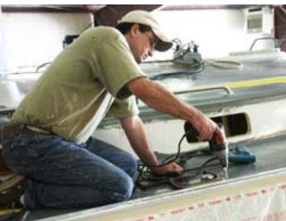
A worker finishes the toe rail. The grey goop protects the deck. It rubs off like rubber cement.
