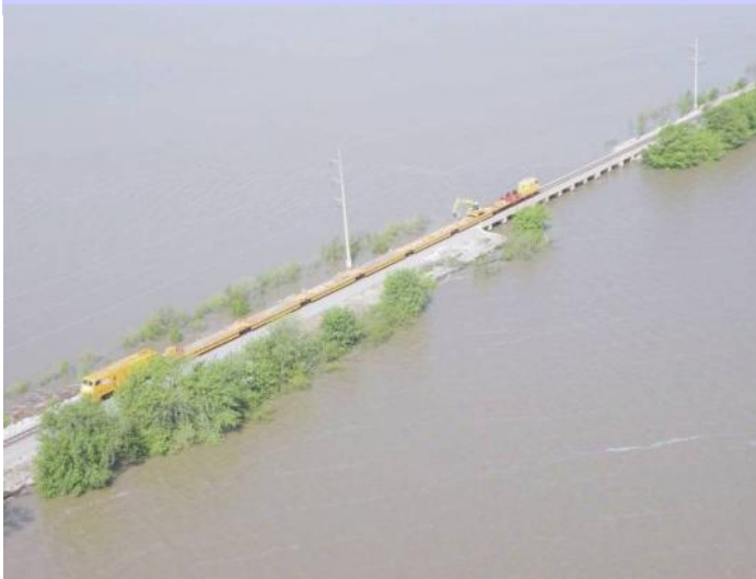
Overhead photo of Burlington Northern Railroad crews adding gravel to fight erosion, May 4th, 2011 - photos provided by the Army Corps of Engineers, Carlyle Lake Management Office
